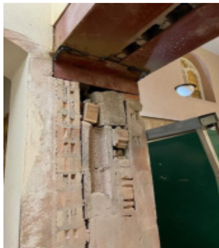
New steel at Miller Center and Heritage Center entry to support headers.
