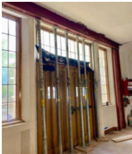
New steel at Miller Center and Heritage Center entry to support headers.
