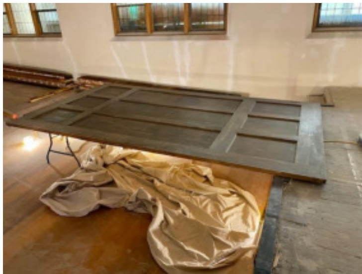
One panel of Heritage Center sliding door, stripped and cleaned.
