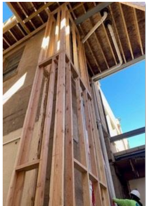
Westminster Commons wall furring, re-routed roof drains
