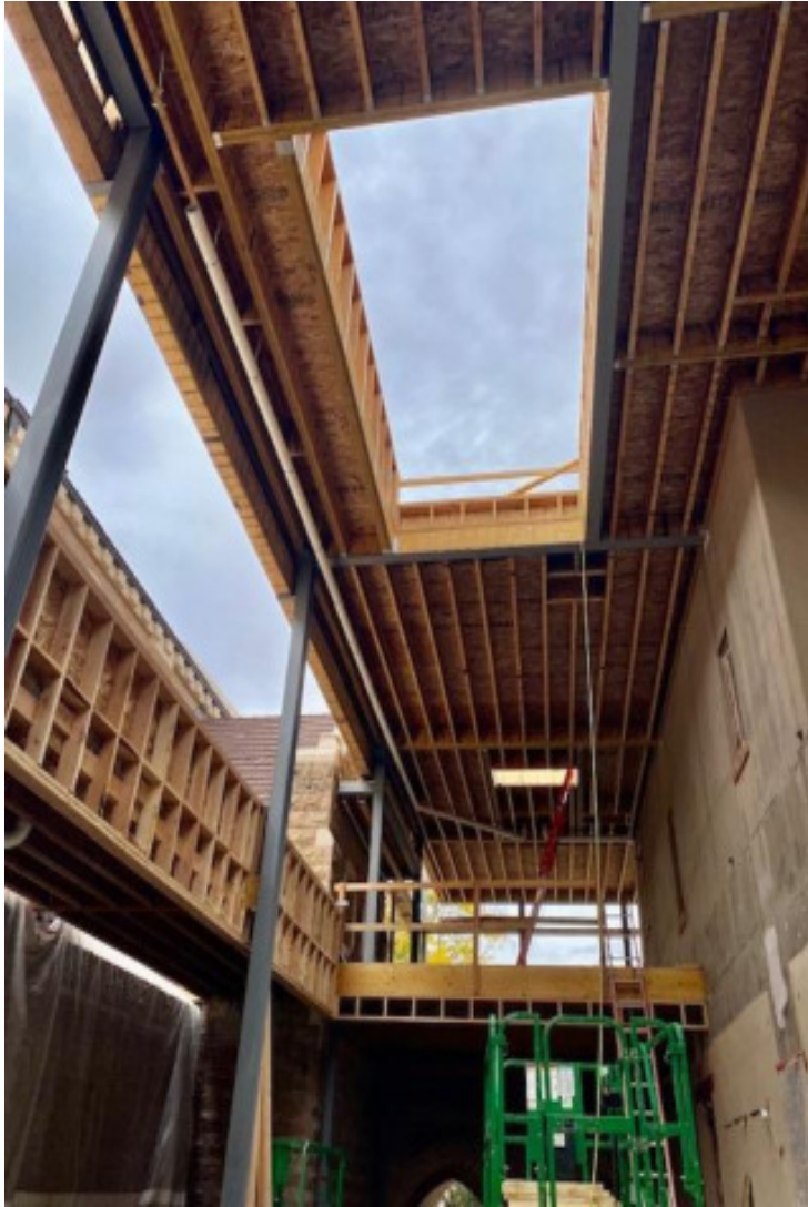
Westminster Commons framing looking towards new bridge
