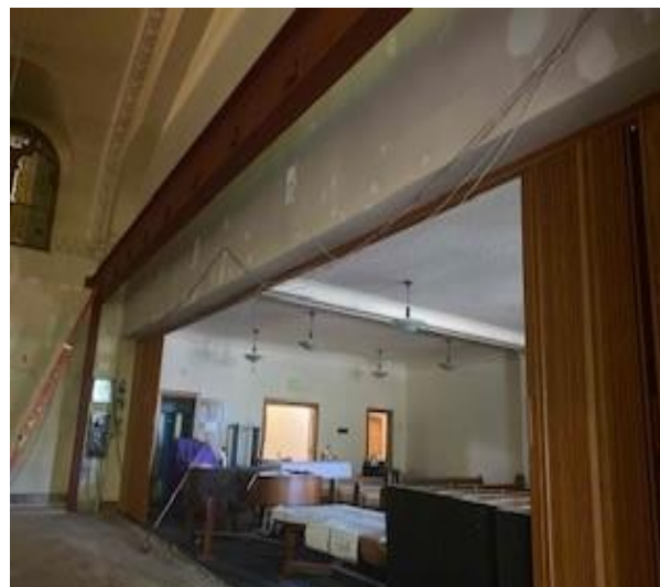
New steel installed
