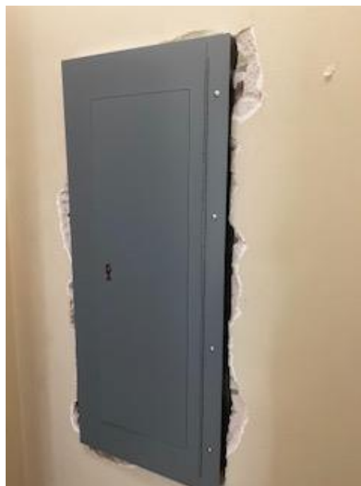
TI electrical panel installed
