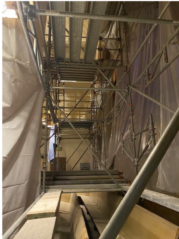
Scaffolding in choir loft.
