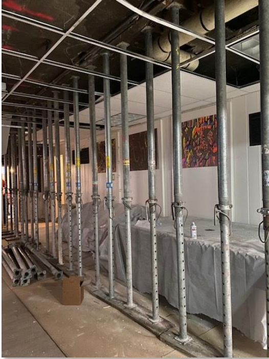
Shoring under Miller Center for new steel
