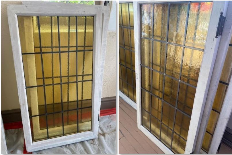
Newly re-built windows for re-installation in Tower.
